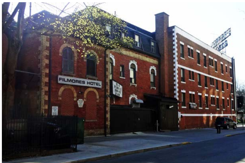
On George Street, north of Dundas Street East, the late 19 th century house form building known historically as the Henry Tasker House is attached to the rear (north) side of the hotel.
